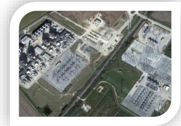
1.2 MW combined cycle Power plant
