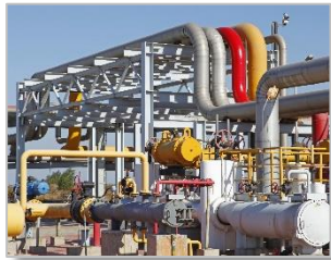
Natural Gas Pipeline Strategic Account Mgmt
